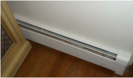
Figure 6. Baseboard radiator (left); radiant flooring (right)
