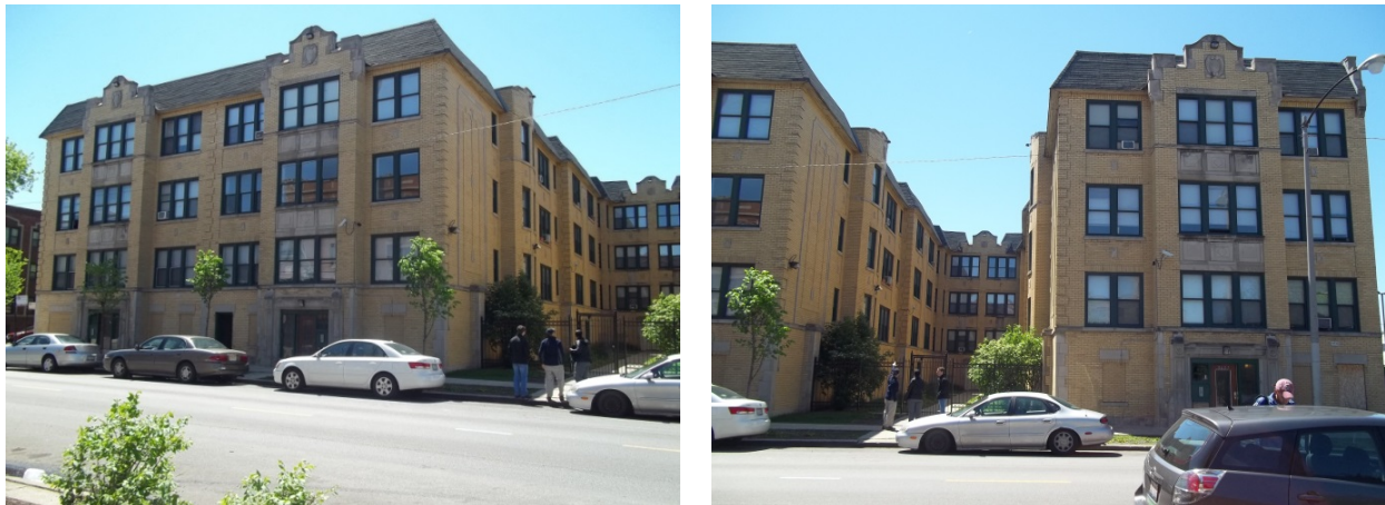
Figure 8. Photograph of Building A: northeast corner (left); northwest corner (right)
