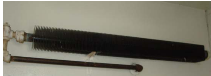
Figure 5. Radiator (top left); convector (top right); finned-tube (bottom)
