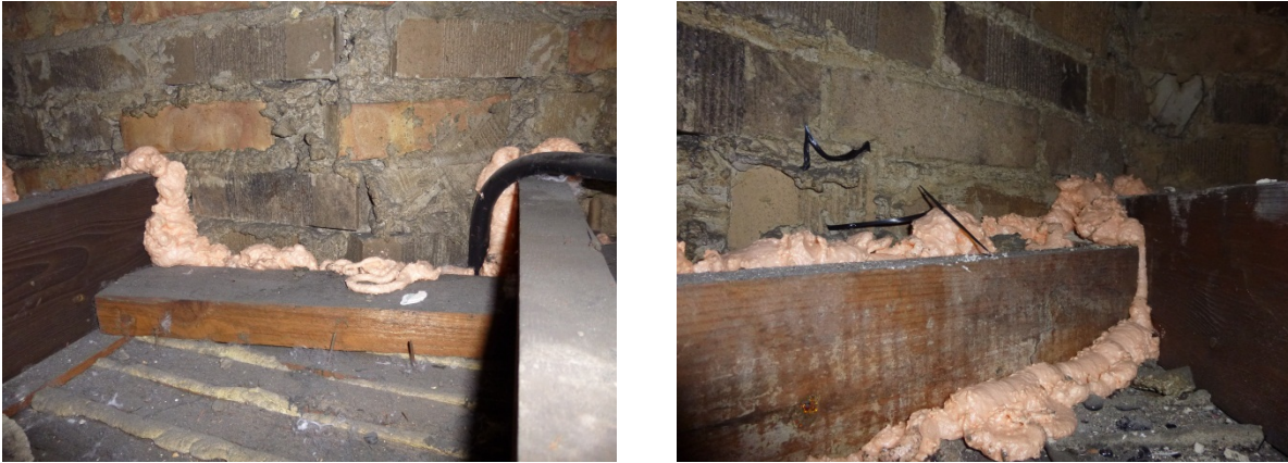
Figure 6. Air sealing around the perimeter of the roof cavity.
