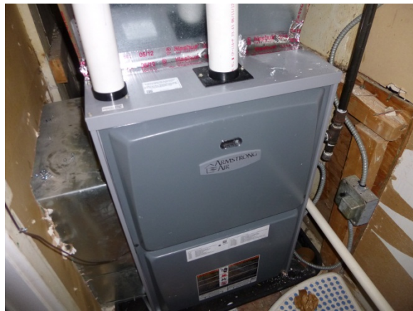
Figure 13. Left: Old furnace. Right: New high efficiency (95% AFUE) furnace with PVC venting.
