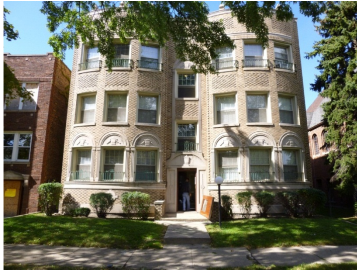
Figure 3. Building 1 from the front entrance.
