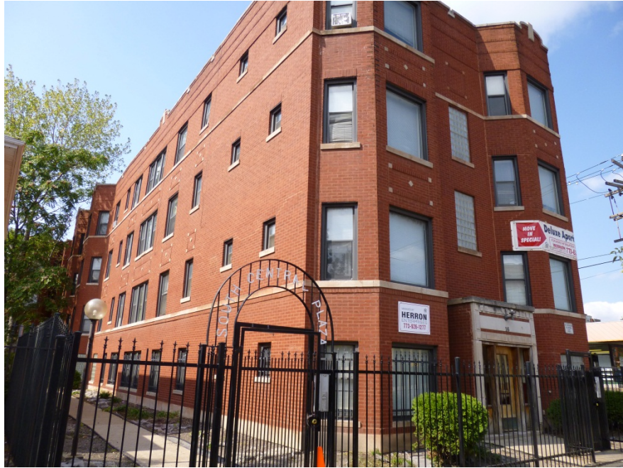
Figure 8. Building 2 from the front entrance.
