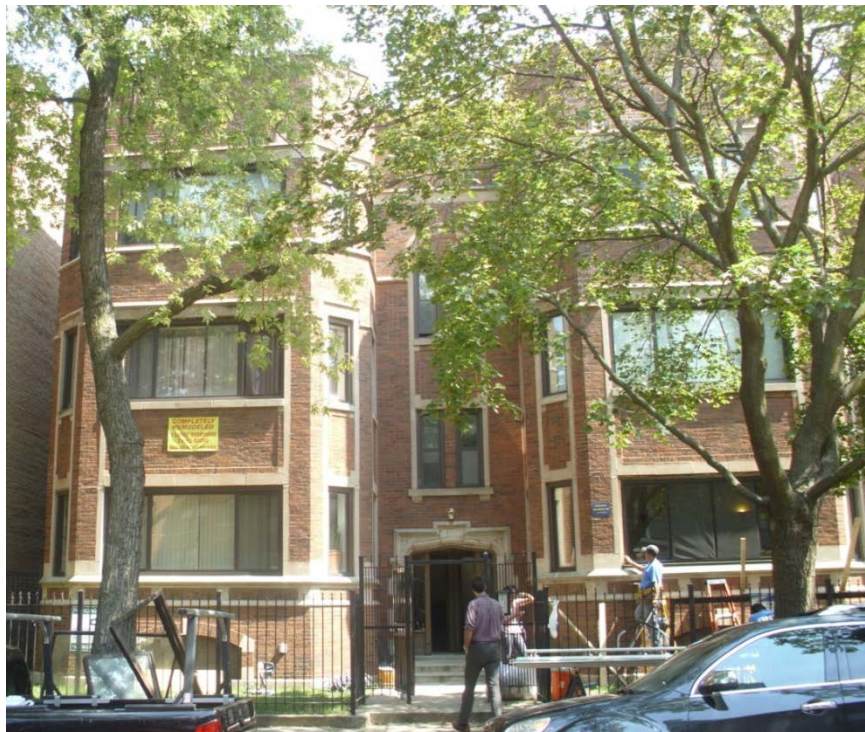
Figure 12. Building 3 from the front entrance.
