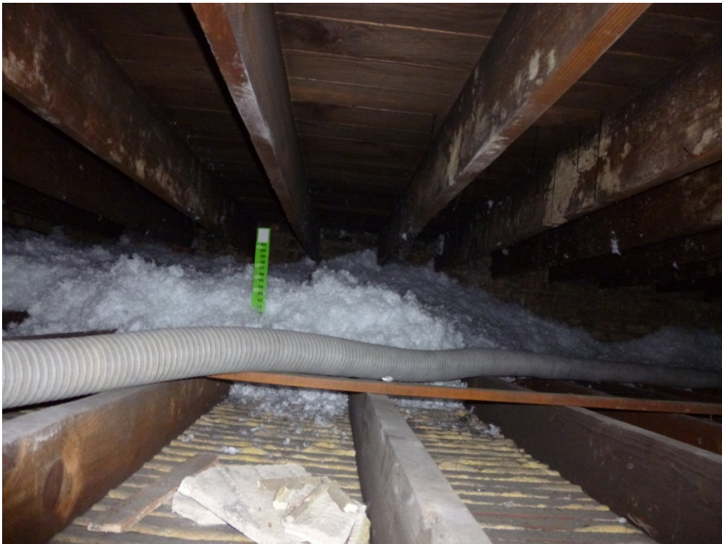
Figure 7. Insulating the roof cavity with loose fill fiberglass.
