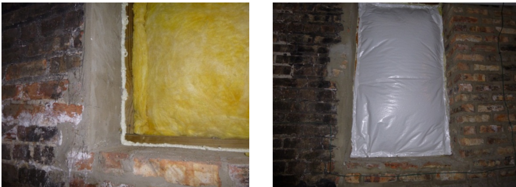
Figure 10. Window opening sealed and insulated with batt insulation.
