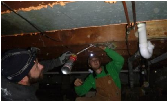
Figure 1. Sealing of abandoned panned return (left); use of rigid foam and sealant to shut abandoned supply boots (right)
