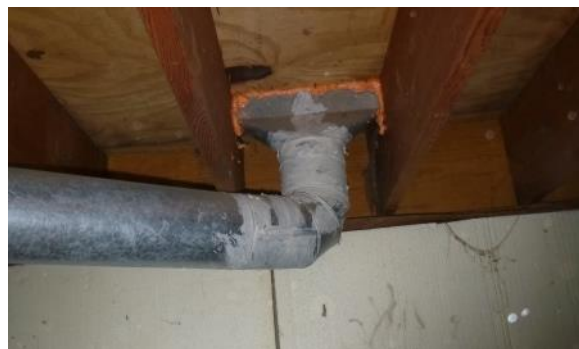
Figure 1. Sealing of abandoned panned return (left); use of rigid foam and sealant to shut abandoned supply boots (right)
