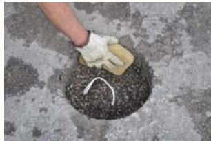
Install Lead and Clean coresd hole
