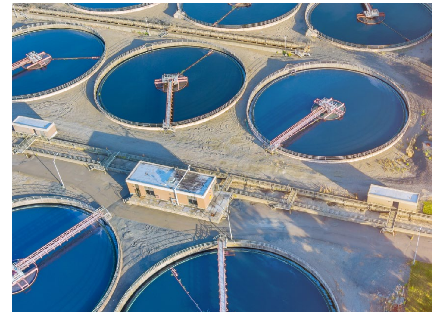
Biogas Conditioning & RNG Upgrading
